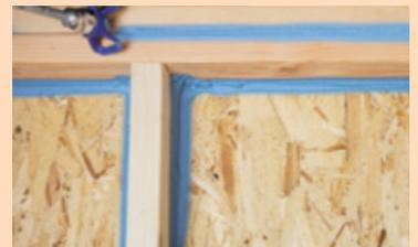
*ECOSEAL Plus™ can be applied to the top plate to form a drywall gasket.*
