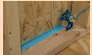
*ECOSEAL Plus™ spray sealant should be sprayed on all joints, gaps and seams prior to insulation.*
